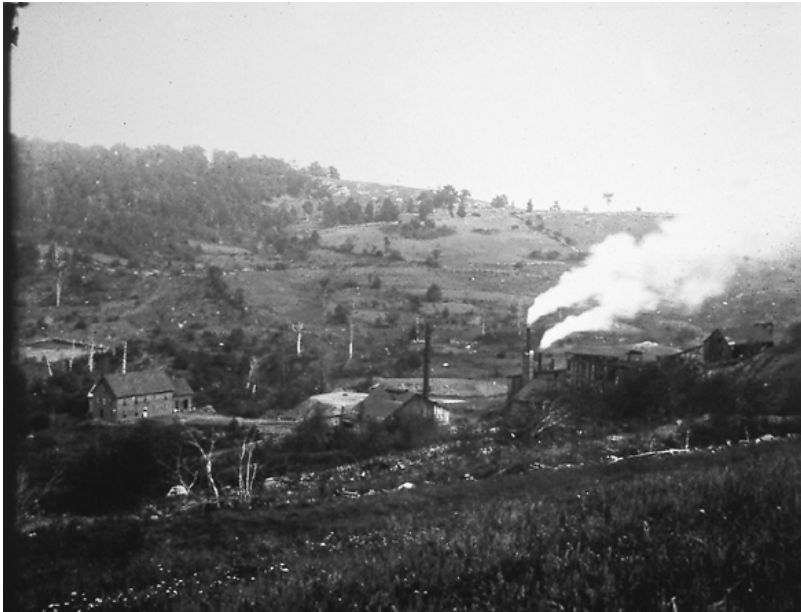
Figure 8. Tyson copper smelter operating, c. 1900 (possibly 1907) with smoke emanating from blower engine and blast furnace stacks. The reverberatory furnace was housed in the structure with the idle smokestack and the building to the far left was a miners' boarding house constructed c. 1900. Photograph courtesy of the Strafford Historical Society.
