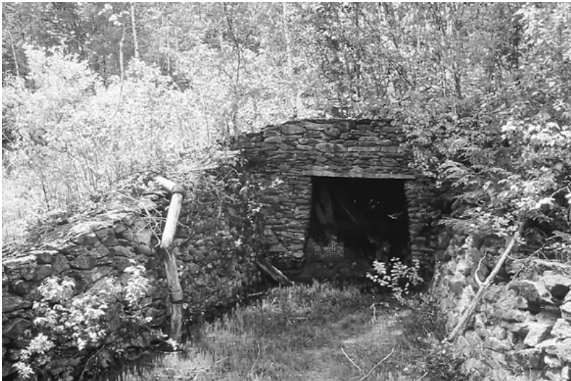
Figure 5. The Tyson Adit (1,340 feet long) was completed in 1898 and served as the mine's main entrance until 1958. June 1994 photograph by the author.
