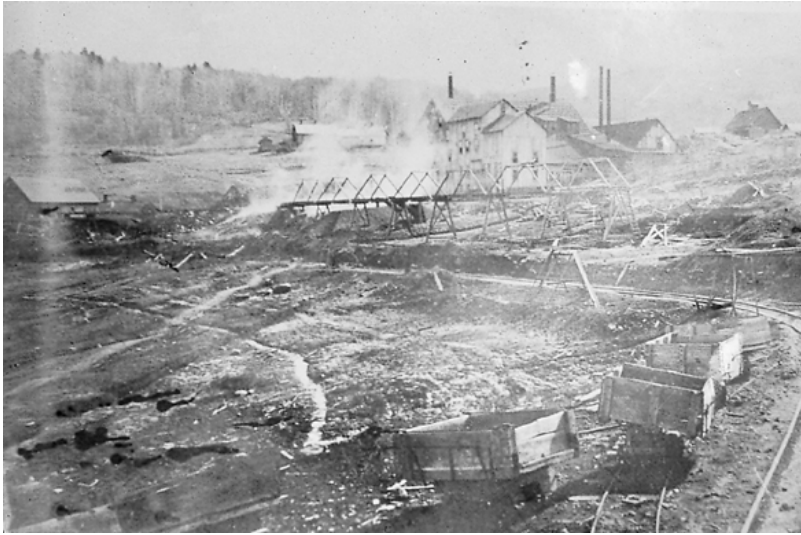
Figure 6. Heap-roasting near the Elizabeth Mill, c. 1902. Smoke from the roast beds near the left end of the railway trestle partially obscures the mill building. The wooden ore cars in the foreground were used to charge the copper blast furnace located near the photographer's vantage point. Collamer Abbott Papers, Special Collections, Bailey/Howe Library, University of Vermont, carton 13, folder 3.
