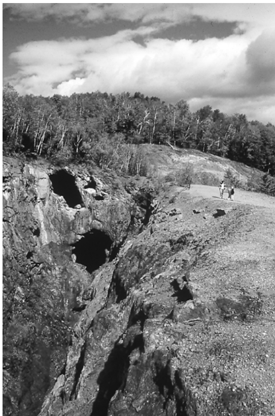
Figure 4. View of the deep Elizabeth Mine north open cut on Copperas Hill from the south. This pit was last mined on the old Foster-Cleaveland tract by the Vermont Copper Company during the 1940s and 1950s, obliterating remnant copperas mining excavations. This final phase exposed old mine openings from the Tyson era where the large ore body dips beneath the surface. The mine and mill buildings from the 1880s were located on the right side of the dumps. October 1998 photograph by the author.
